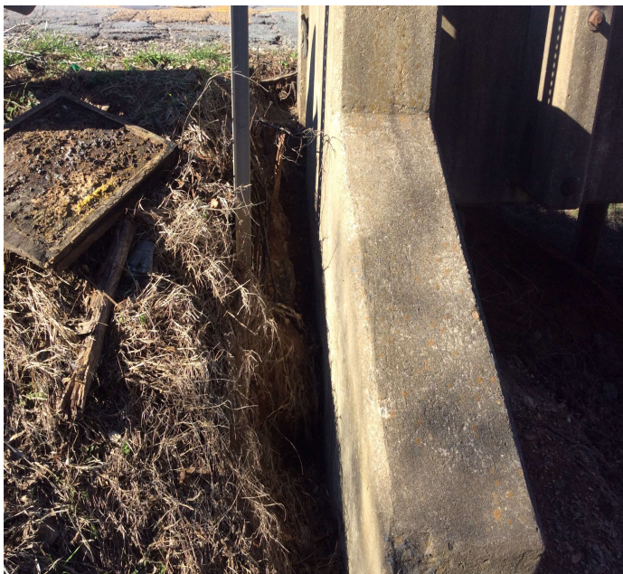
PHOTO 1 Description Abutment - Bent 1 right (erosion)
