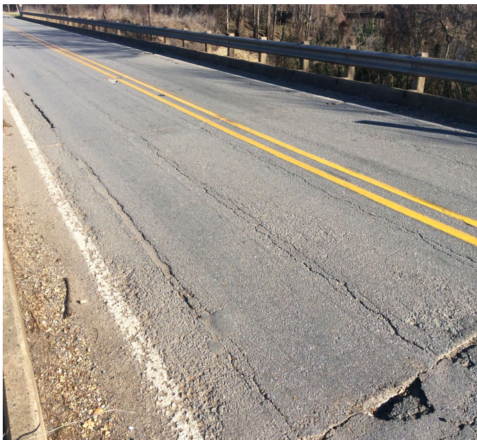
PHOTO 1 Description Asphalt wearing surface - Spans 1-2 (deterioration)
