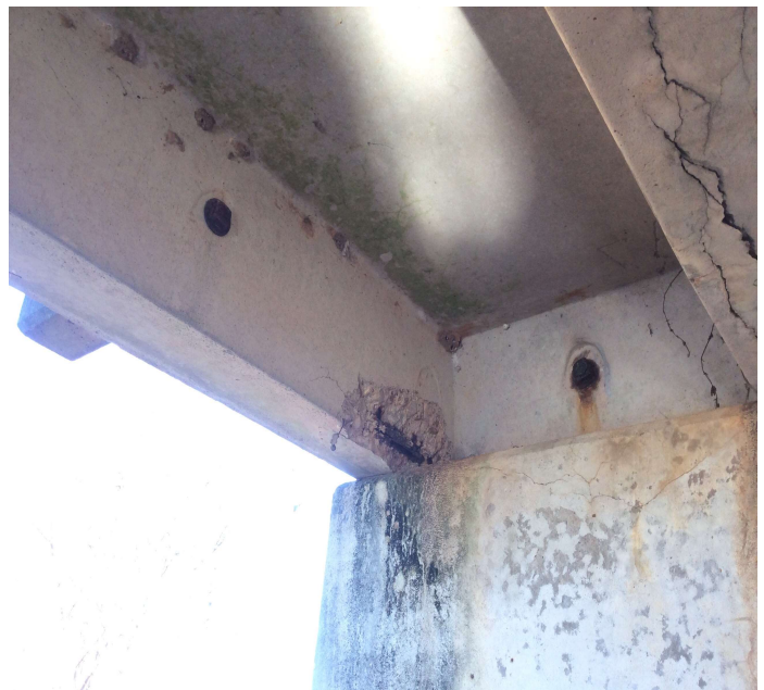
PHOTO 2 Description Span 12 Unit 1 @ Bent 13 (rebar exposed)
