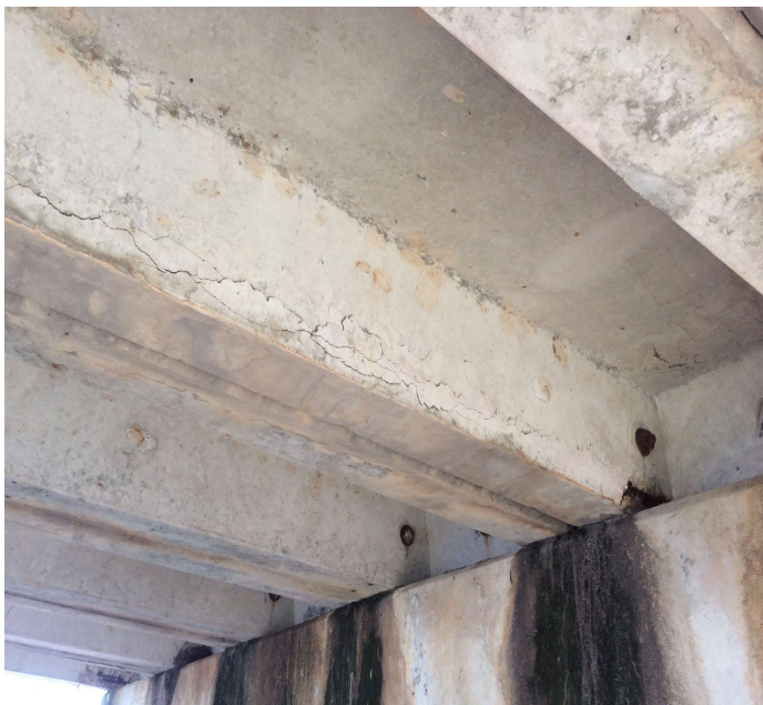
PHOTO 1 Description Span 12 Unit 5 @ Bent 13 (rebar exposed/cracking/delaminating)
