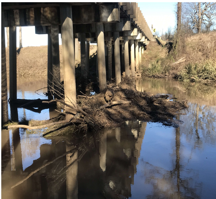
PHOTO 4 Description Debris field at piles bents 6-8.
