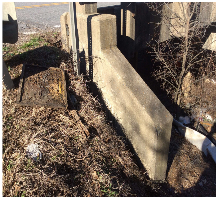
PHOTO 2 Description Abutment - Bent 1 right (erosion)
