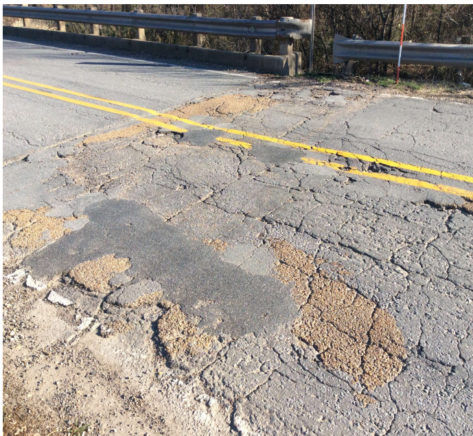
PHOTO 1 Description Approach roadway - Bent 1 (deterioration)
