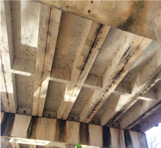
PHOTO 3 Description Span 10 Unit 4 (rebar exposed)
