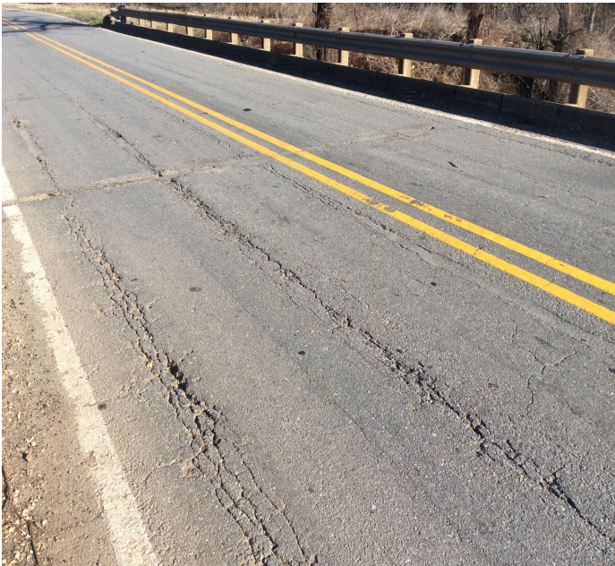
PHOTO 2 Description Asphalt wearing surface - Spans 9-10 (deterioration)
