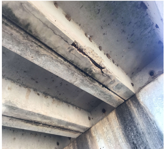
PHOTO 6 Description Span 12 unit 1 girder legs have spalls with exposed rebar. Common unit 5 this span.
