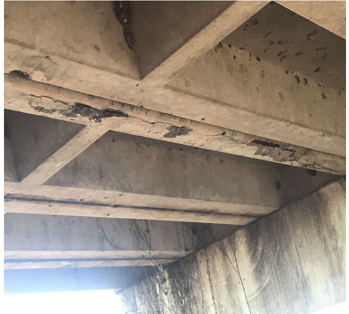
PHOTO 5 Description Span 2 girder 3 spalling to channel legs.
