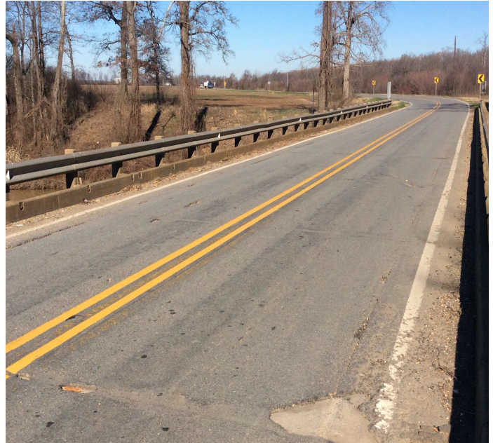
PHOTO 3 Description Asphalt wearing surface - Spans 4-5 (deterioration)
