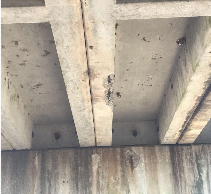
PHOTO 7 Description Span 2 girder 6 has spalling to channel legs.
