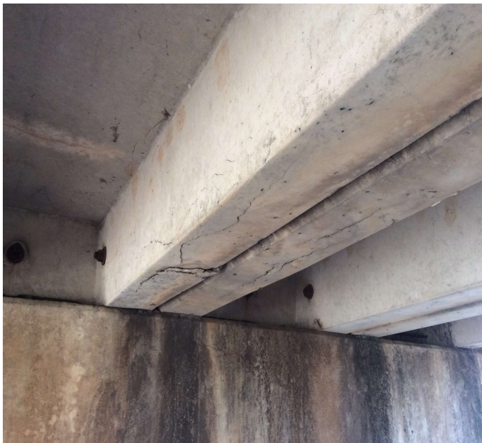
PHOTO 1 Description Span 13 Units 3-4 @ Bent 13 (cracking/delaminating)
