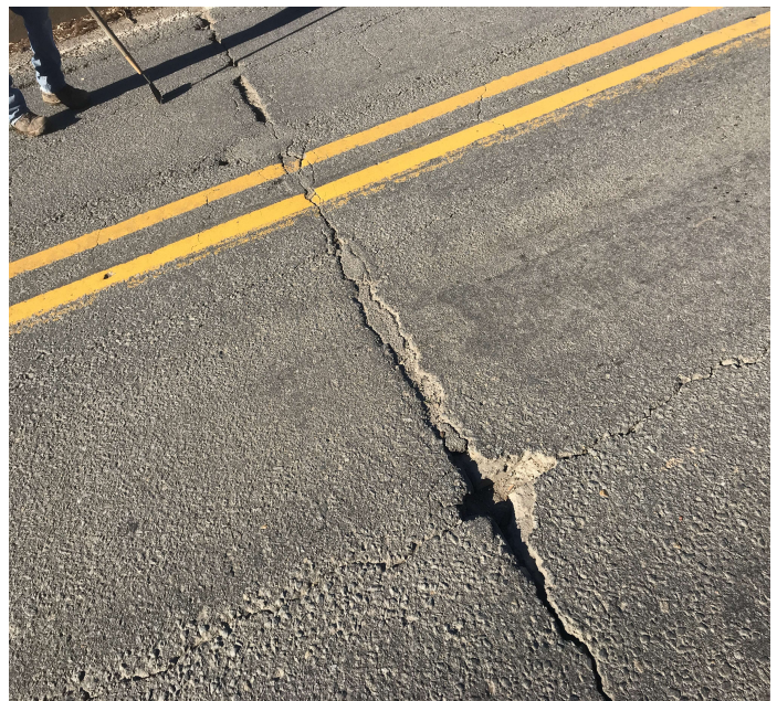
PHOTO 1 Description Deck all spans have small spalls in asphalt wear surface at unit ends and key ways.
