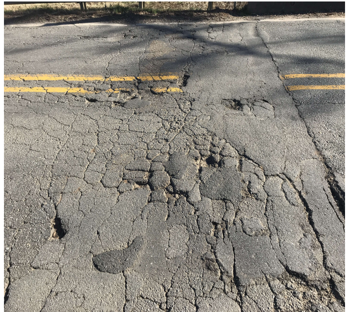
PHOTO 3 Description Bent 14 approach roadway has small pothole in asphalt.
