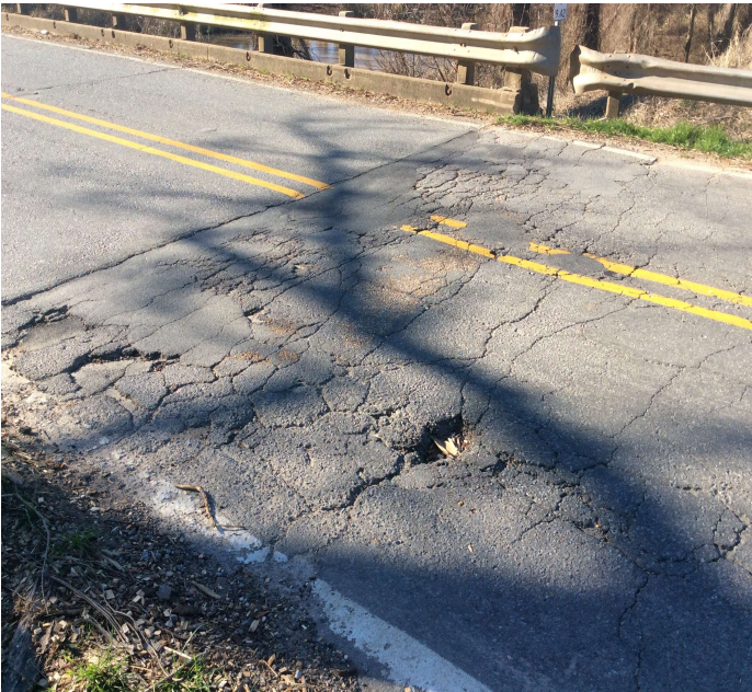
PHOTO 2 Description Approach roadway - Bent 14 (deterioration)
