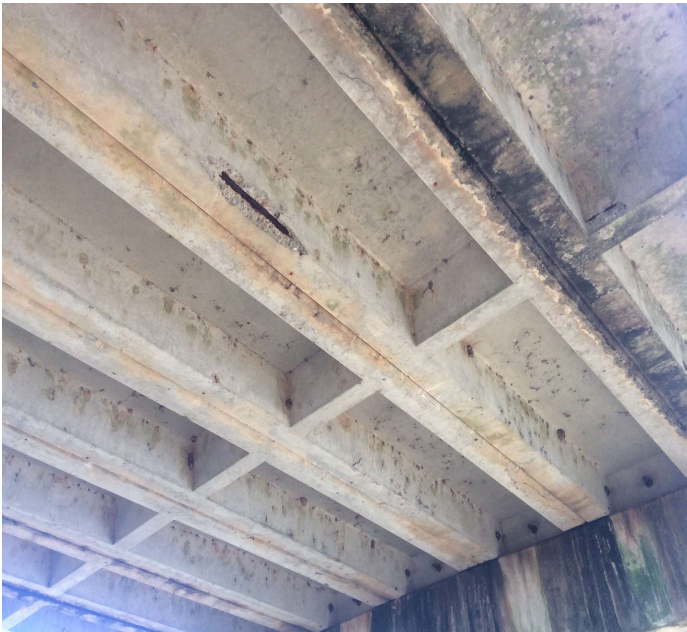
PHOTO 4 Description Span 4 Unit 6 (rebar exposed)
