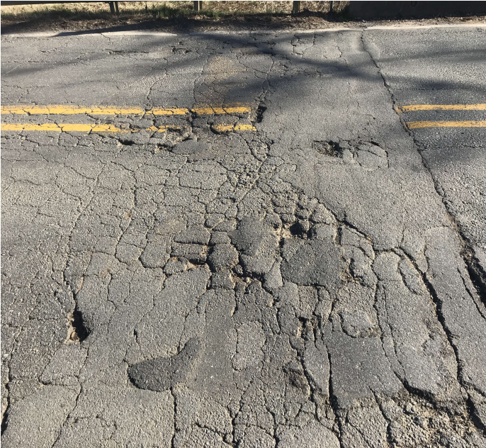
PHOTO 2 Description Bent 14 approach roadway has small pothole in asphalt.
