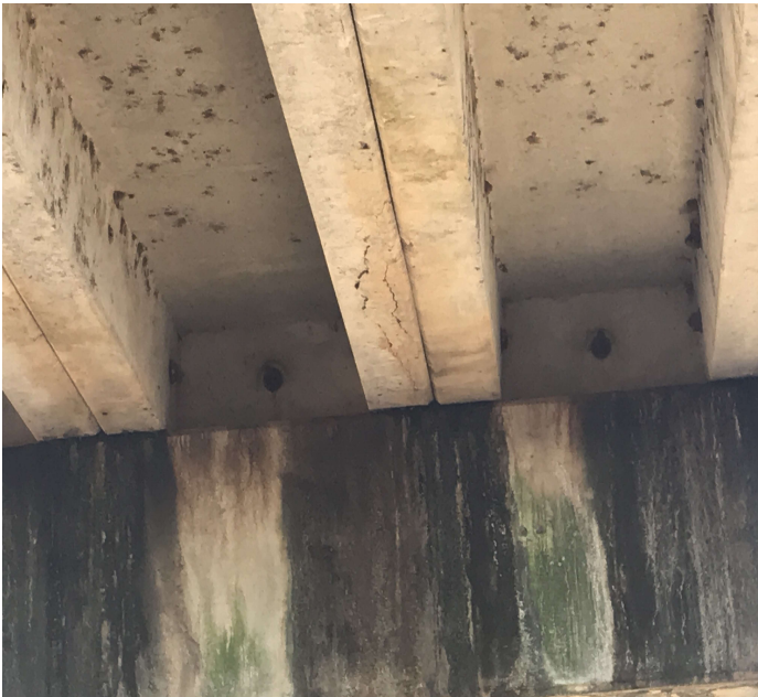
PHOTO 8 Description Span 4 girder 5 has cracks and delam in channel legs. Common girder 3 this span.
