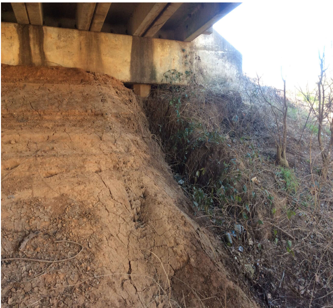
PHOTO 1 Description Endslope - Bent 1 left (erosion)
