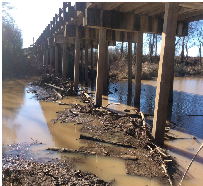
PHOTO 1 Description Channel - right side (debris build-up)
