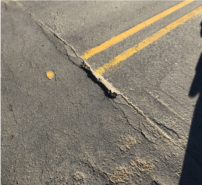
PHOTO 2 Description Bent 1 approach roadway has small pothole near centerline.
