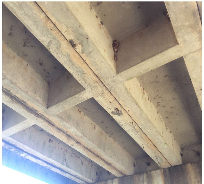
PHOTO 2 Description Span 2 Unit 3 (cracking/delaminating)
