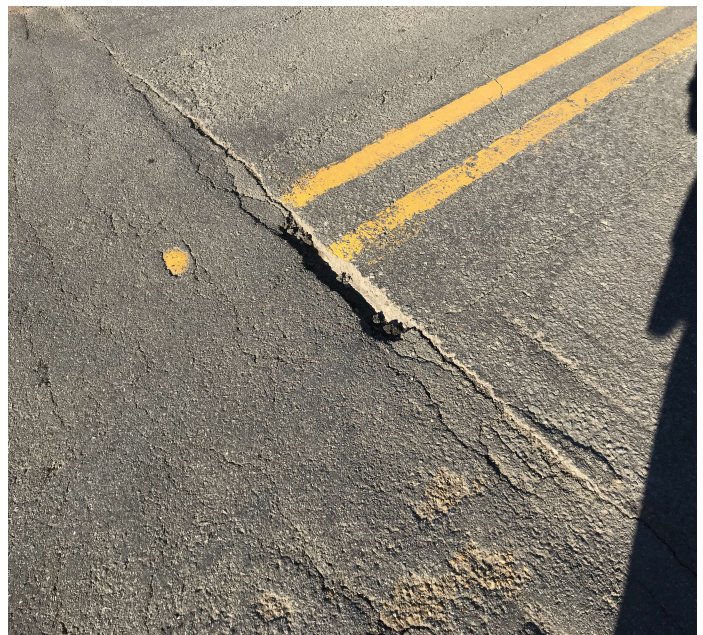
PHOTO 1 Description Bent 1 approach roadway has small pothole near centerline.
