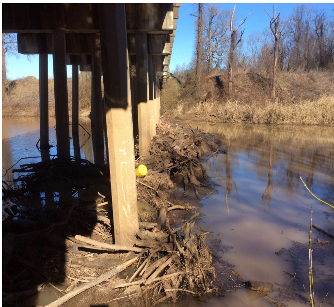
PHOTO 3 Description Channel - right side (debris build-up)
